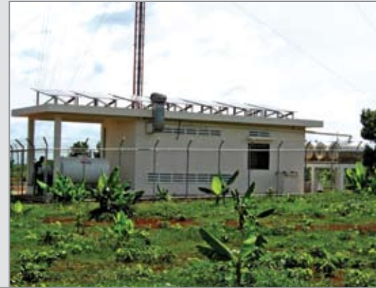
GSM Base Station Installation Location: Cambodia System Size: 3.36 kW
