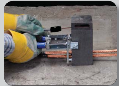
step 3 • Attach cord to UltraShot™ igniter
