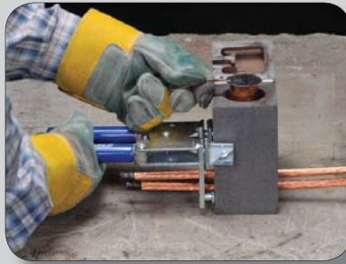
step 2 • Close handle clamp and lock mold • Insert UltraShot™ drop-in into mold
