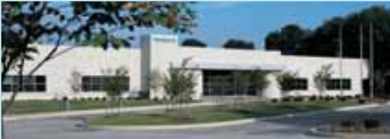
GLOBAL LOGISTICS CENTER / MARYLAND
